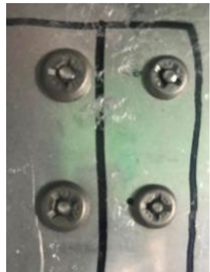
Fig. 2- Typical example of Installed Blind-Bolt Fasteners
