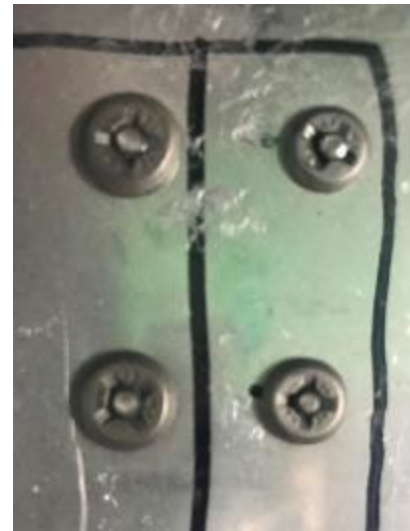
Fig. 2- Typical example of Installed Blind-Bolt Fasteners
