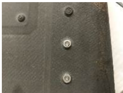
Fig 3- Installed Blind Rivets with Coating Removed
