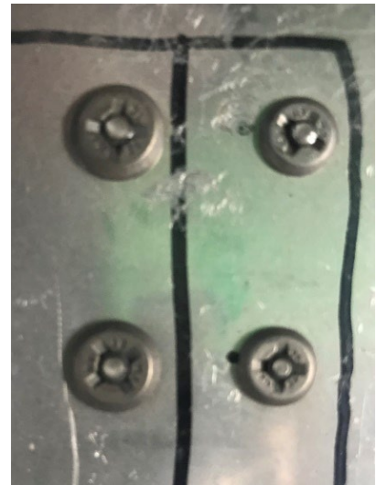
Fig. 2- Typical example of Installed Blind-Bolt Fasteners
