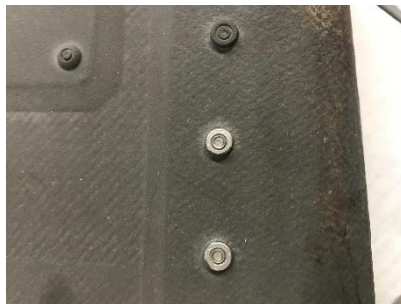
Fig 3- Installed Blind Rivets with Coating Removed
