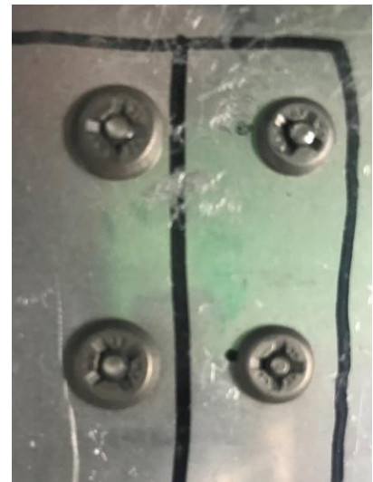
Fig. 2- Typical example of Installed Blind-Bolt Fasteners
