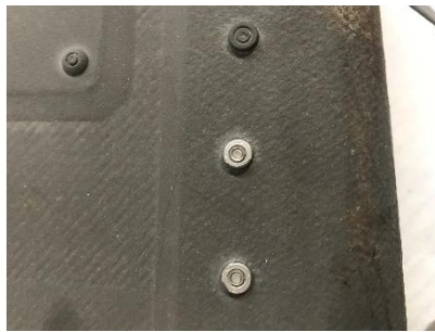
Fig 3- Installed Blind Rivets with Coating Removed
