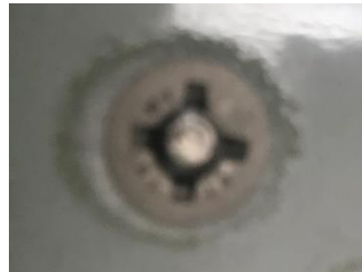
Fig. 3- Typical example of installed Blind-Bolt with coating removed
