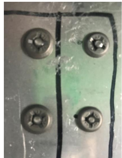
Fig. 2- Typical example of Installed Blind-Bolt Fasteners
